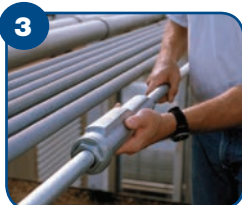
3 Thread the next length of conduit into the other end of the fitting and tighten. You're done!
