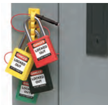
5. Low-profile lockouts allow panel doors to be closed on most breaker panels.
